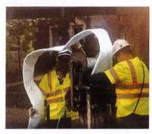
SJCM Approach & Advantage: Our team members inspected 18" CIPP installation for the Port of Oakland. As a first order of work, SJCM RE will set up a special meeting with the Contractor and the CIPP subcontractor to go over all the critical steps. An agenda will be prepared that would address the following issues:
